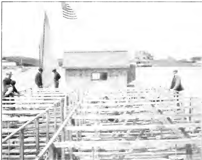
VIEW OF REARING PLANT AT WOODS HOLE, SHOWING METHOD OF TRANSMITTING POWER TO THE FANS.
