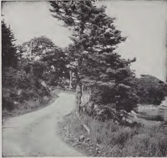
Good Roads Wind Along the Rivers Among the Pines and Spruces
