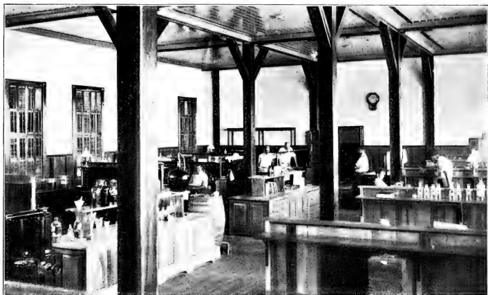
LABORATORY INTERIOR, BEAUFORT.
