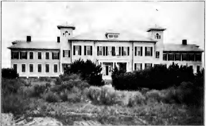
BEAUFORT LABORATORY—EXTERIOR VIEW.
