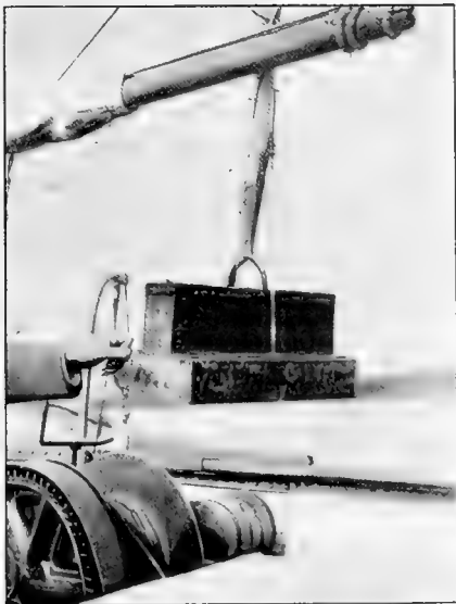
Fig. 1. Earlier apparatus with pole, to take up 1 square foot of bottom-soil.
