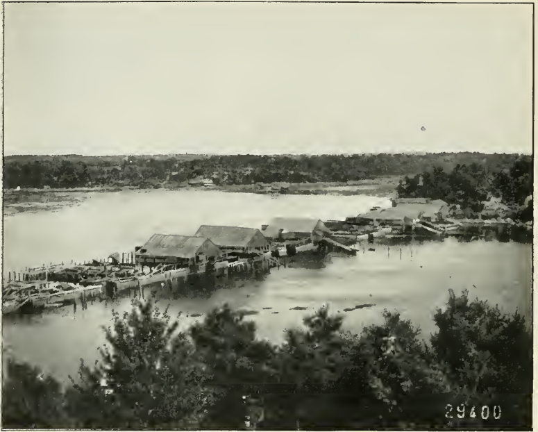
Old tide water saw mills, first started in 1833
