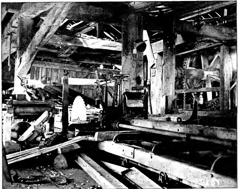
View inside one of the old tide mills still running. Shows rotary saw and carriage (modern) old windlass wheel for hauling logs out of the water; and edger.
