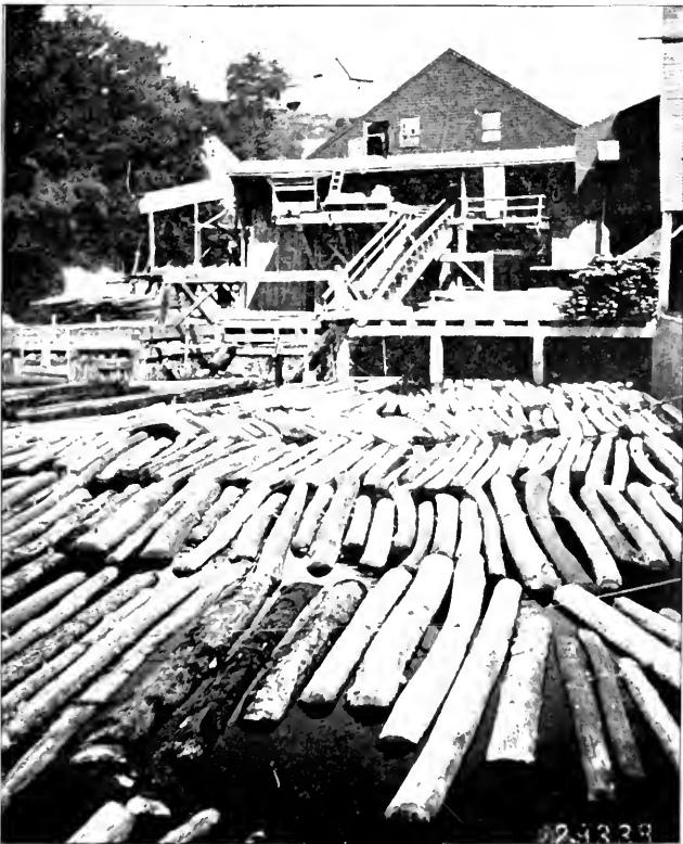
Log pond slip, Bangor
