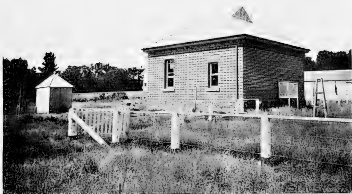
ANOTHER VIEW OF THE ADELAIDE SEISMOGRAPH HOUSE.
