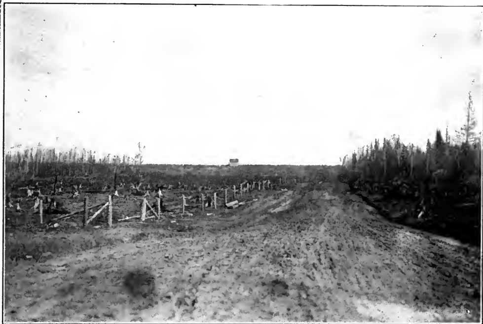
A Trunk Road one mile north-east of the Town of Cochrane, showing the Taylor Farm.
