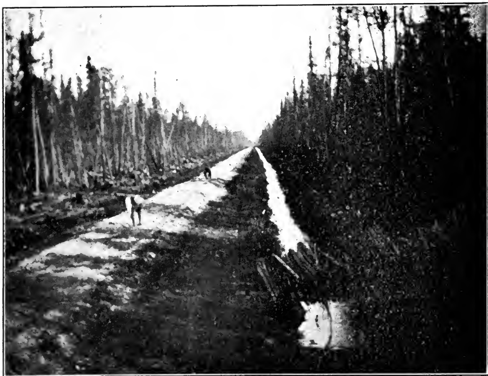
Surfacing a Semi-Muskeg Road with Gravel. Part of the Little Grassy River Road, Rainy River Valley.
