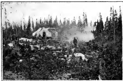
Burning off the right of way on the trunk road west of Cochrane.
