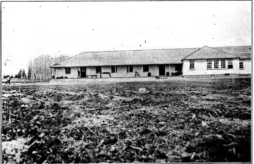
The Fort William and Duluth Trunk Road passing the Provincial Government's Prison Farm, south-west of Fort William.
