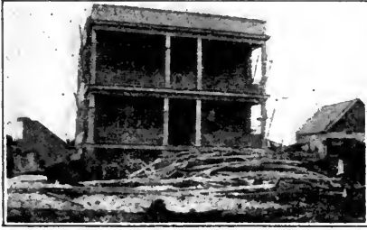
Transcontinental office building at Hearst.
