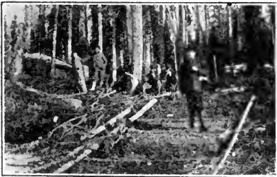
A road cut-out, south boundary of Glackmeyer.
