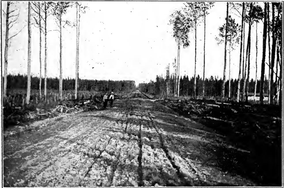
On the Town Line between Glackmeyer and Lamarche, east of Cochrane, showing how Clay Roads are rutted during the wet season.
