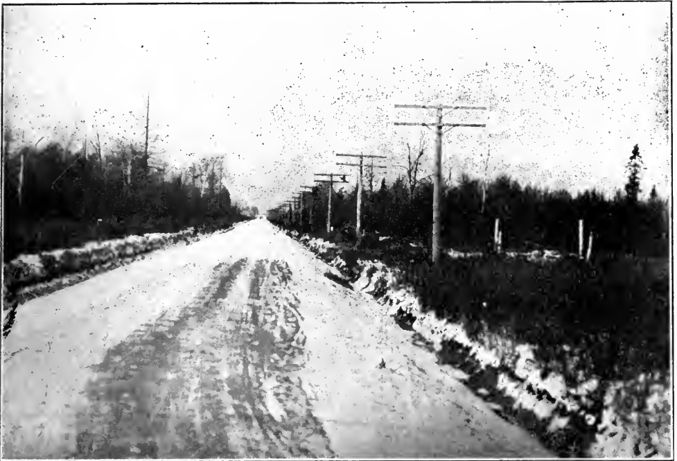
View of the Macadamized Road east of Sault Ste Marie, on the Sudbury and Sault Ste. Marie Trunk Road.
