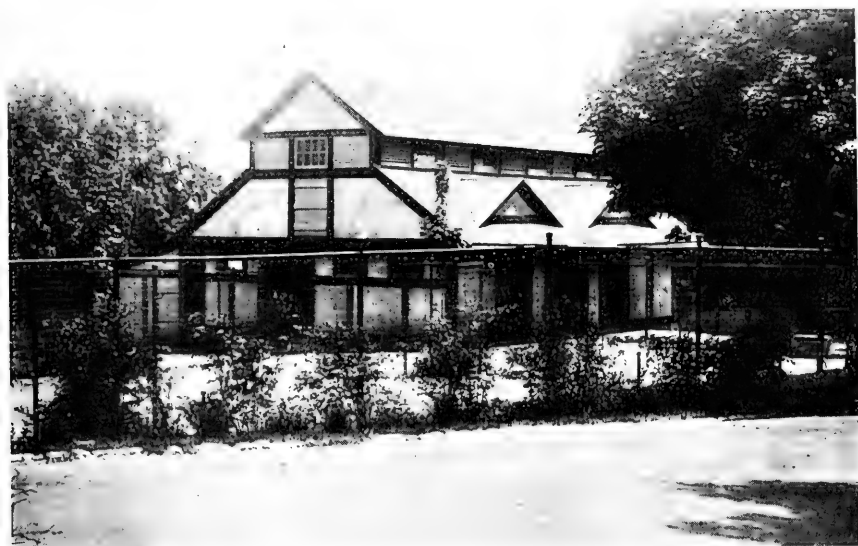
FIG. 1.—THE RECONSTRUCTED BUFFALO HOUSE, NOW USED AS A SHELTER FOR THE MOUNTAIN SHEEP, ELANDS, AND KASHMIR DEER, RECENT GIFTS TO THE PARK FROM CANADA AND ENGLAND.
