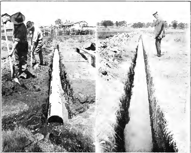
b. Laying 10 inch corrugated pipe Gourley Tract, Stamford.
