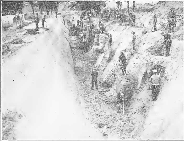
FIGURE 96. Laborers excavating a deep main ditch from East Hartford meadows to Connecticut River.
