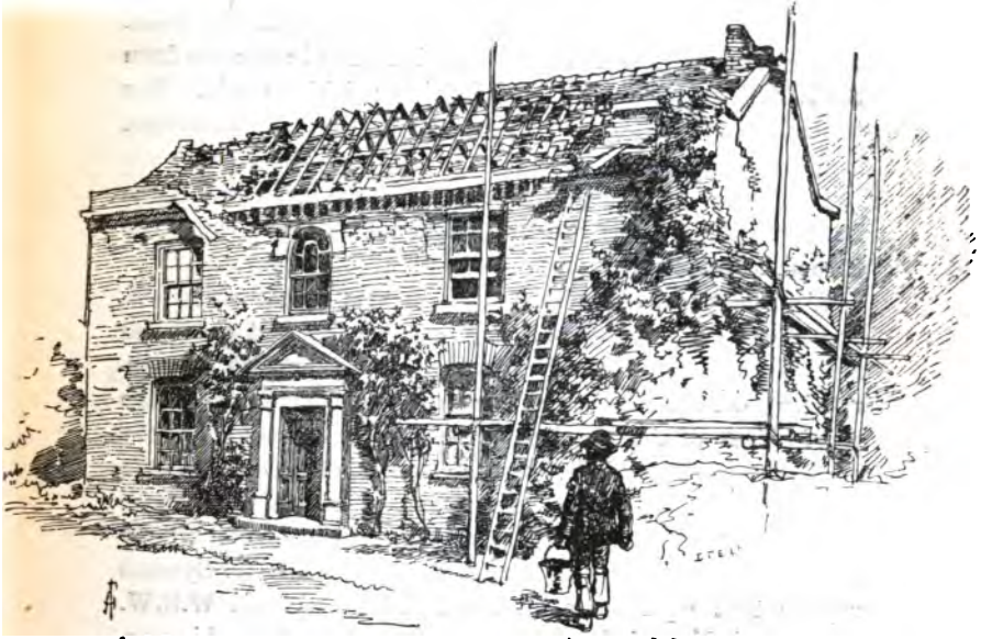
FIG. 8.—Brick House, Great Wigborough.
