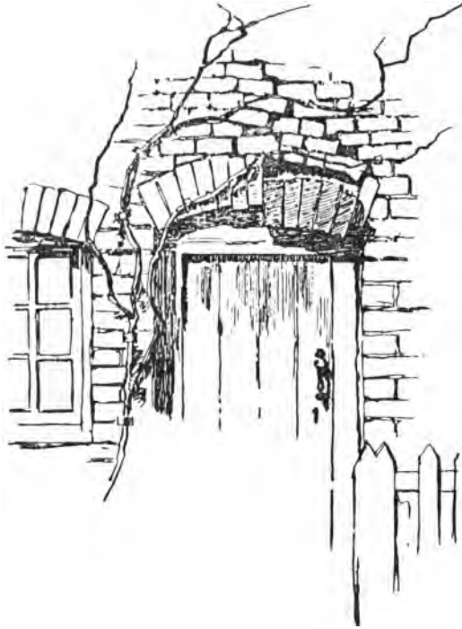
FIG. 11.—Doorway at Peldon, showing loosened bricks.
