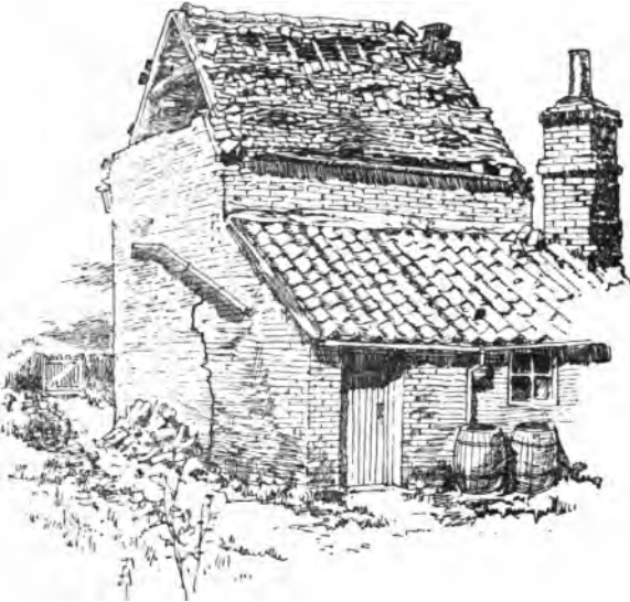
FIG. 5.—Shattered Cottage at Peldon.
