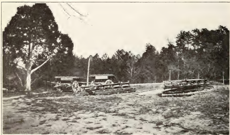
FIG. 2.—WAGON BEDS USED FOR MOVING CAMP AND SECTIONS OF BUILDINGS.
