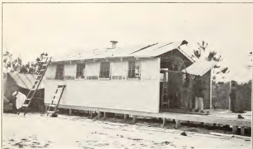
FIG. 1.—TEARING DOWN BUILDING BEFORE MOVING EXPERIMENTAL CAMP.
