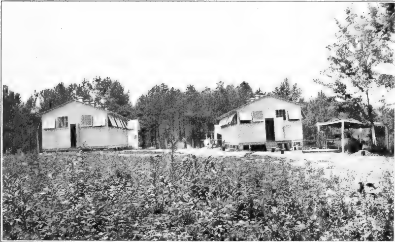
FIG. 2.—PORTABLE QUARTERS OF THE GEORGIA CAMP. DESIGNED TO ADMIT ABUNDANT LIGHT AND AIR.
