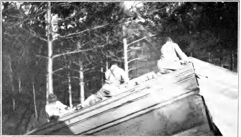
FIG. 2.—PUTTING ON ROOF STRIPS AFTER MOVING EXPERIMENTAL CAMP.
