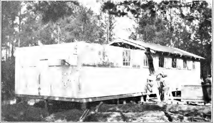
FIG. 1.—PLACING ROOF ON BUILDINGS AFTER MOVING EXPERIMENTAL CAMP.
