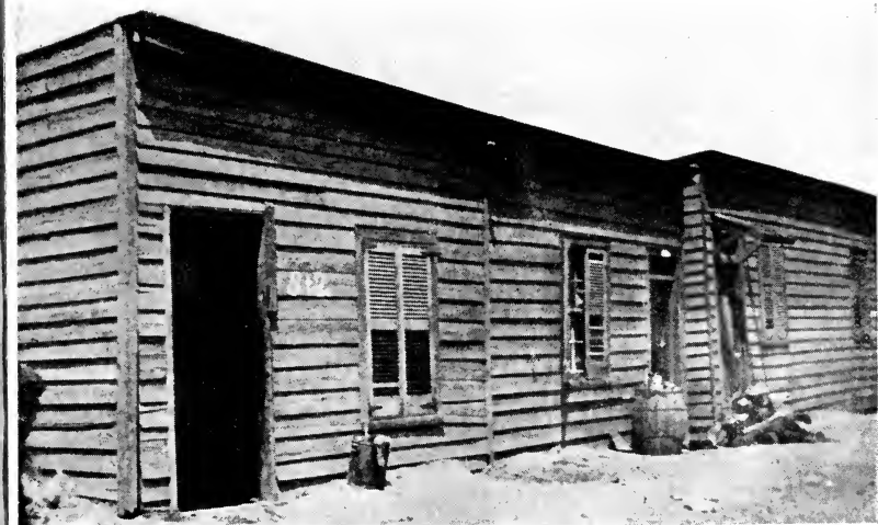
Negro dwellings in the neglected sections of Richmond. These are unfit for habitation.
