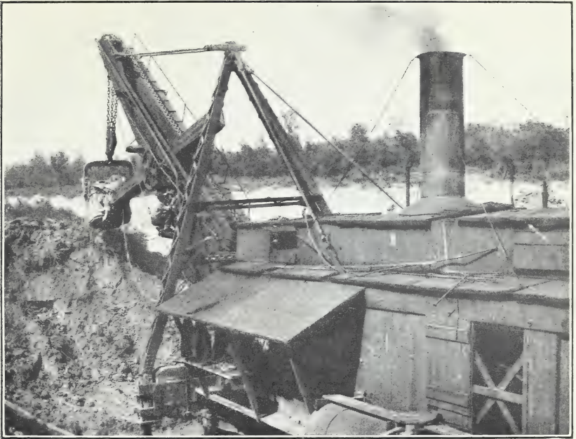
FIG. 1.—MACHINE MINING. REMOVING OVERBURDEN WITH STEAM SHOVEL.
