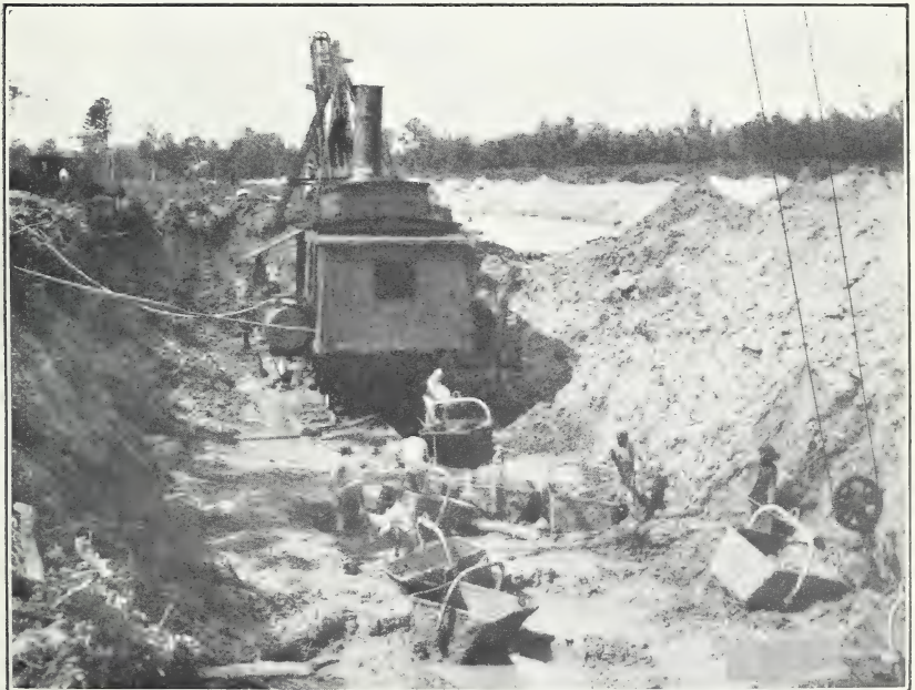
FIG. 2.—LOADING UNWASHED PHOSPHATE INTO BUCKETS TO BE HOISTED ONTO FLAT CARS.
