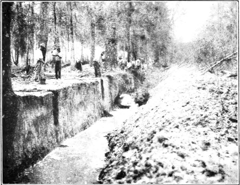
FIG. 1.—HAND MINING. REMOVING OVERBURDEN FROM SOUTH CAROLINA PHOSPHATE.
