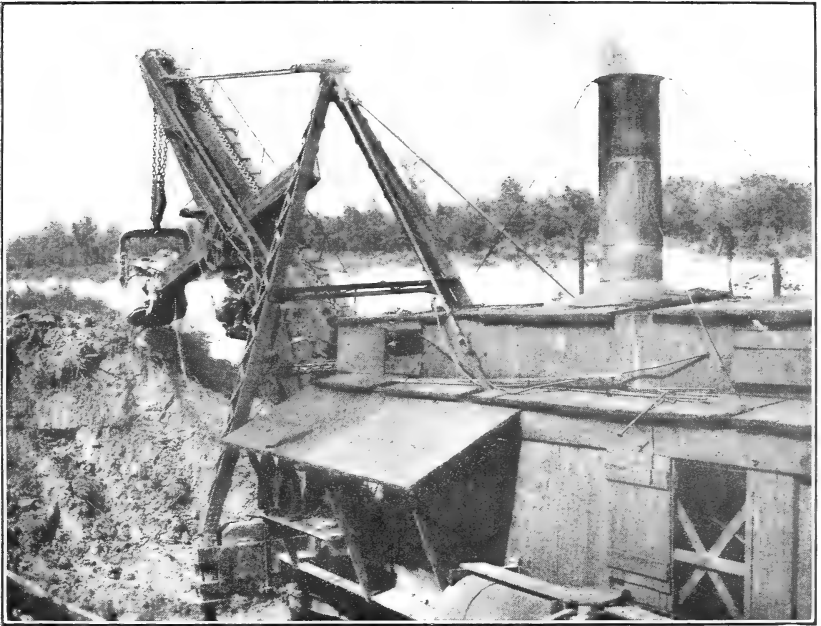
FIG. 1.—MACHINE MINING. REMOVING OVERBURDEN WITH STEAM SHOVEL.
