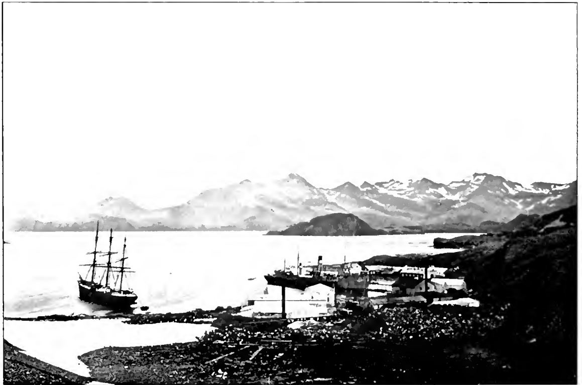
FIG. 2.—Whale Factory, Leith Harbour, South Georgia.
