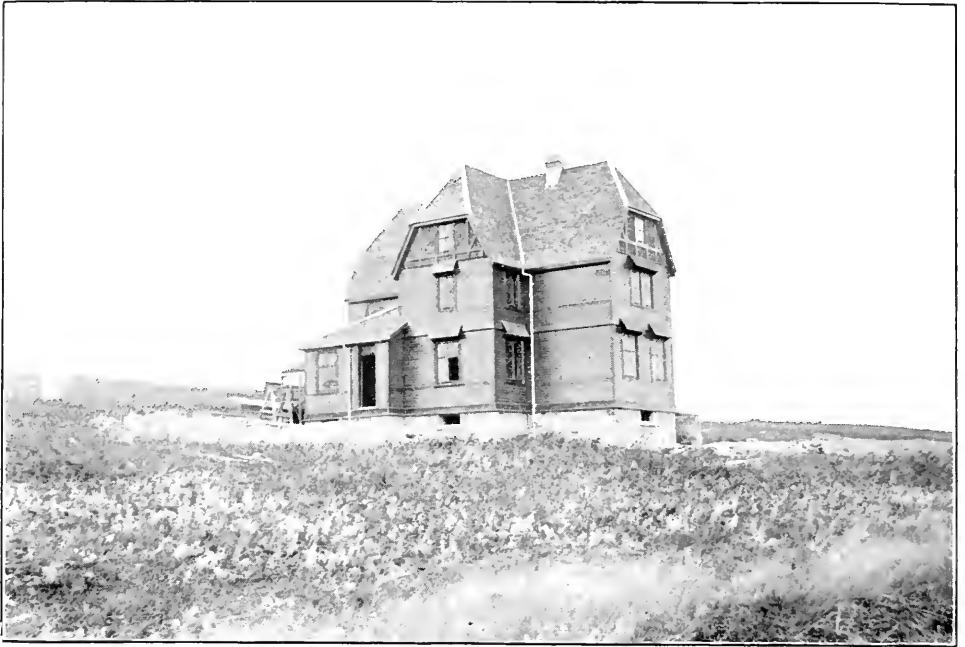
Appearance of grounds surrounding house of Superintendent, Experimental Farm Brandon, Manitoba, at time of building.
