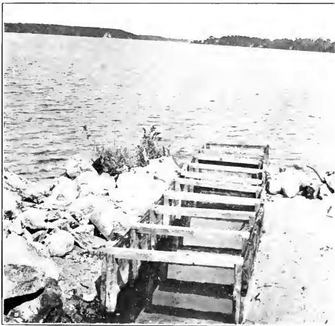
FIG. 2. — Wooden runway at outlet, Long Pond, Harwich.
