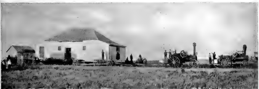
HOUSE MOVED BY TWO TRACTION ENGINES AND EIGHT WAGGONS TWENTY MILES ACROSS THE PRAIRIE FROM WARMAN TO SASKATOON
