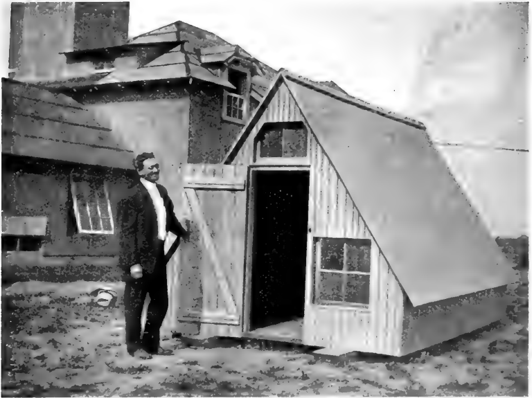
POULTRY HOUSE AT MACDONALD COLLEGE
