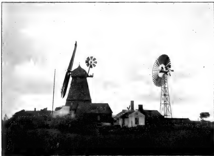
WIND-DRIVEN ELECTRICAL STATION AT ASKOV
