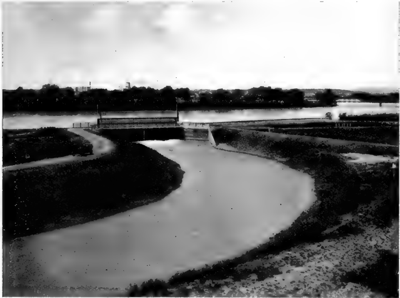
HEADGATE OF IRRIGATION SYSTEM, NEAR CALGARY
