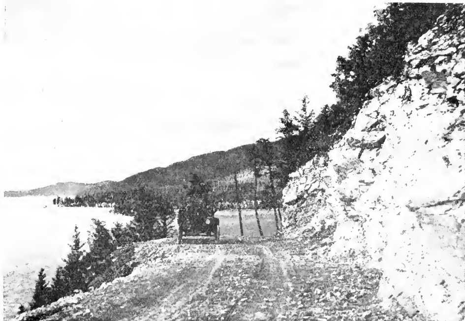
Road Along Shore of Flathead Lake.
