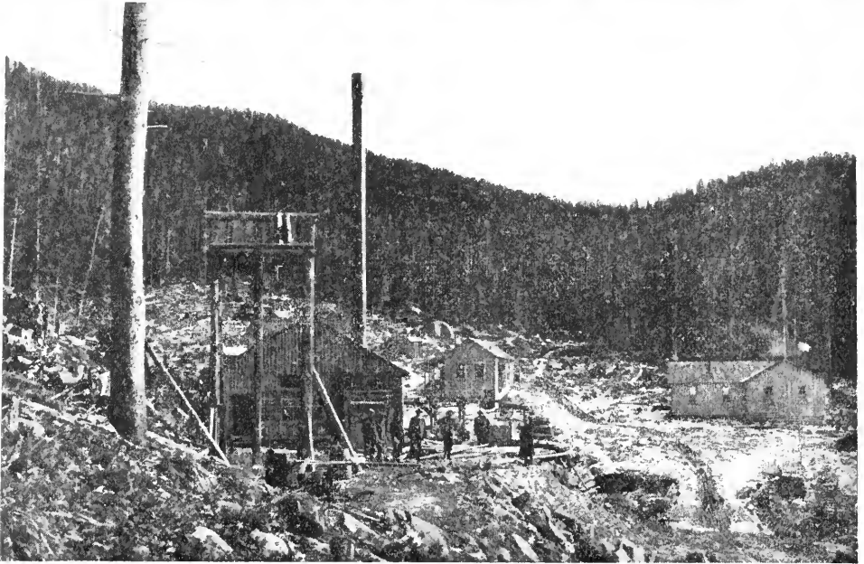
A New Mine in the Forest.
