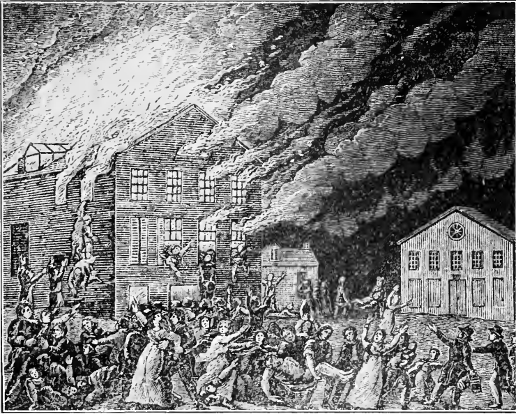
The Burning Theatre, Showing the First Baptist Church to the Right.
