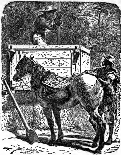
Moulding Brick for Constructing Adobe Buildings.
