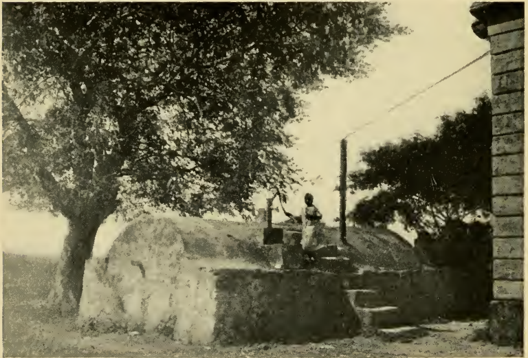
A cistern in which rain water is stored for drinking purposes
