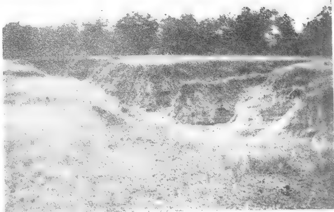
Flooded the barrow pit on the opposite side of road, and poured into farmer's field, leaving a deep wash as a monument.
