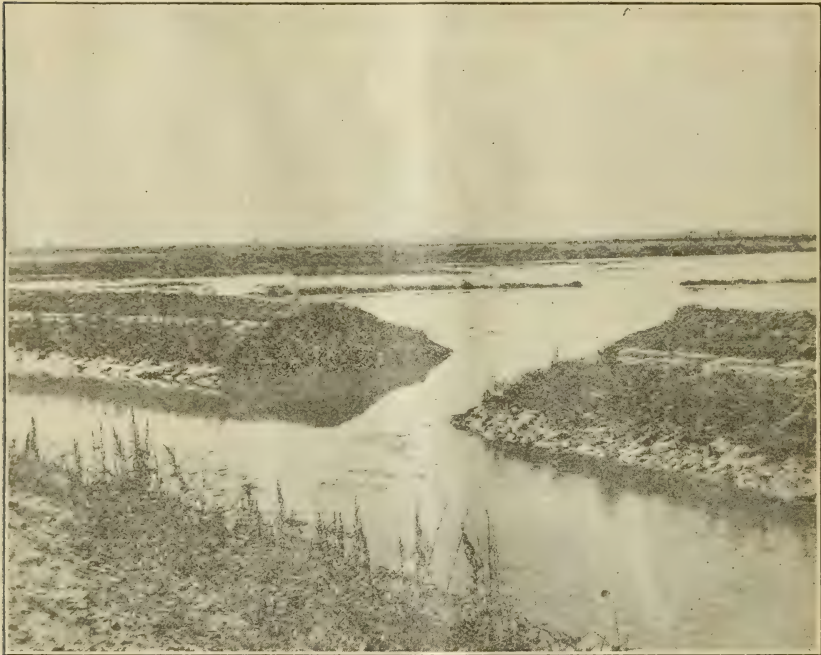
FIG. 10.—Break in irrigation ditch (lateral) caused by burrowing of California ground squirrel. Six acres of alfalfa ruined.
