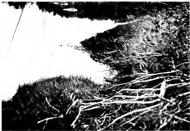
A gate or spillway cut in the dam in order to let the surplus water escape. In times of drought this would be either partly or completely closed.
