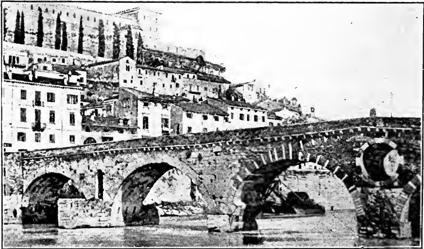
Verona, Augustan Bridge (medieval restorations on right)
