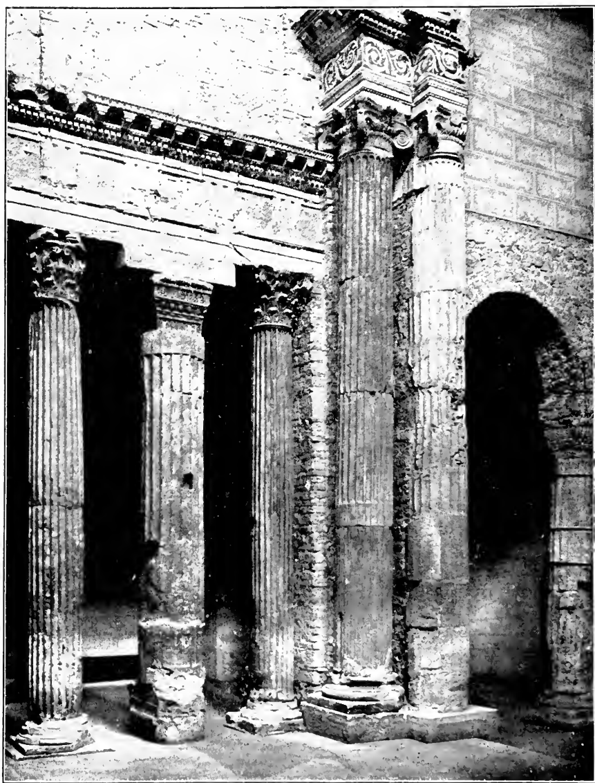
Spoleto, Interior of the Church of the Crocifisso showing profuse and confused use of Roman material
