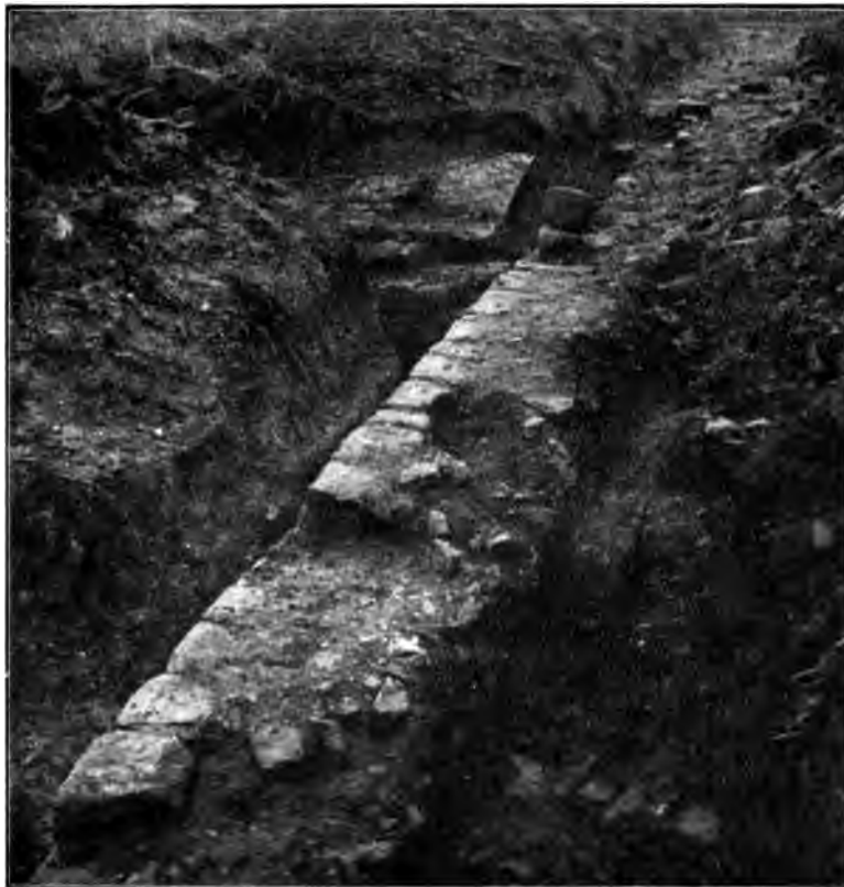
Fig. 12. E. Wall of Praetorium, with remains of Paving, looking N.
