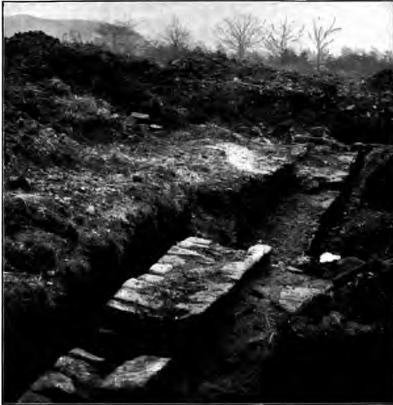
Fig. 13. Partition Wall in Praetorium, showing subsidence on line of Agricolan Ditch.
