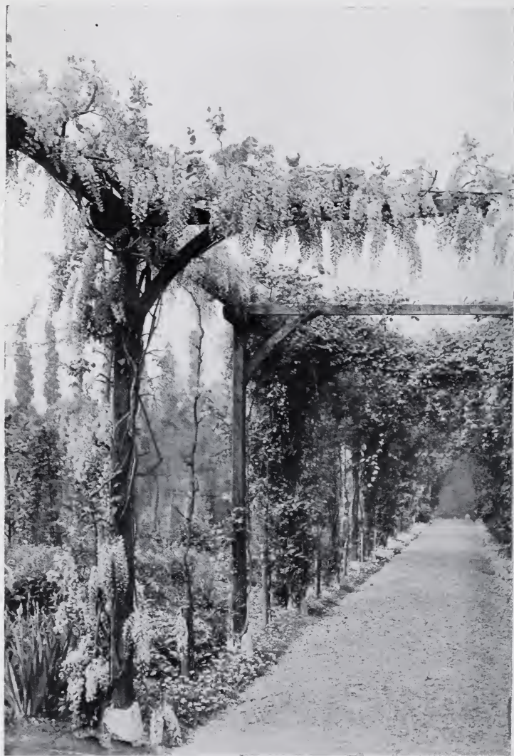
PERGOLA OF LIGHT SQUARED WOOD POSTS ON STONE BASES.
