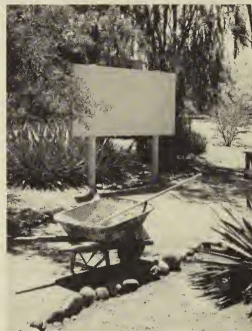
Work in progress on the Demonstration Garden includes new pathway and sign in front of Archer House, as well as laying out the Garden itself.
