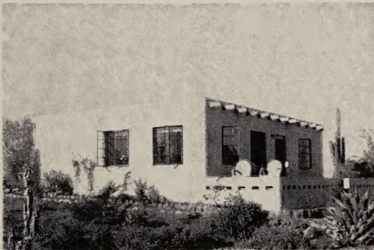
A view of Archer House taken in the summer of 1954 when we added the terrace in front of the residence.
