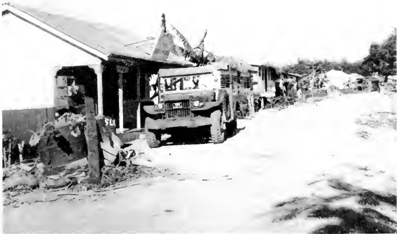
FIG. 11. Tanapag village. Upper: Church. Lower: Street.
