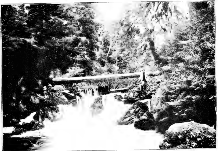
OBSTRUCTION AT KLAKAS, FROM BELOW
