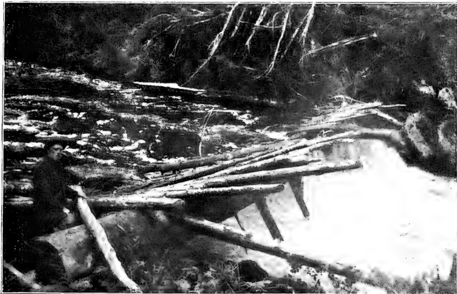
BARRIER IN SALMON STREAM AT HEAD OF HOURS BAY
