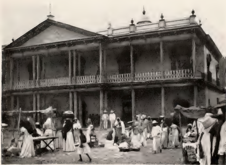
BARRACKS AT COJUTEPEQUE, DEPARTMENT OF CUSCATLÁN.
