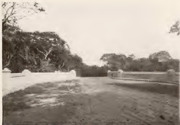
THE NATIONAL ROAD LEADING TO LA LIBERTAD, SHOWING "EL ROTULO" BRIDGE.
