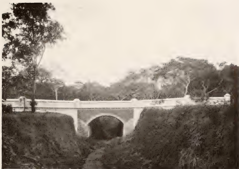
SIDE VIEW OF "EL ROTULO" BRIDGE
