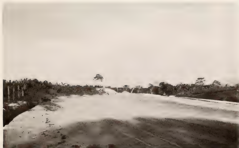
THE FAMOUS AVENIDA UNDER CONSTRUCTION.
