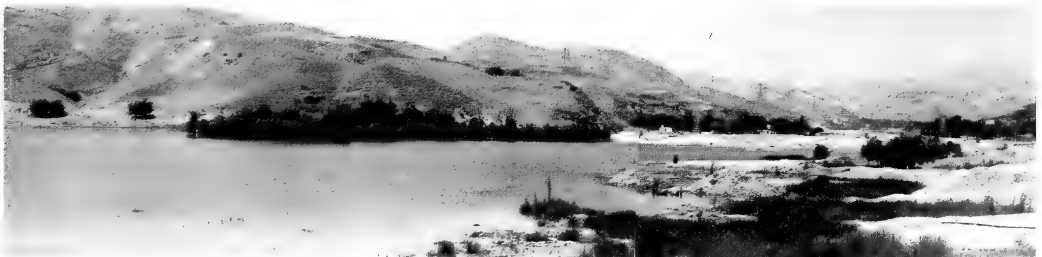
Plate 6. Western part of the Latian Dam, and marshes. © Abolghasem Khaleghizadeh
