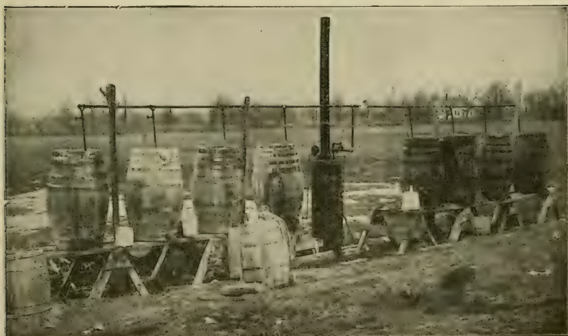
FIG. 2.—Cooking lime-sulfur wash with steam.
