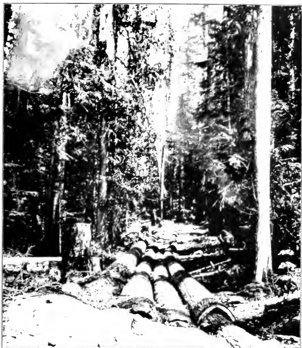
A Douglas Forest in British Columbia. The Skid-way completed.
