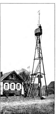
Fig. 289.—Russian watch tower for fire-guard.
