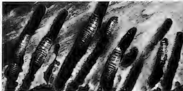
Wood girders bore into a piling.
