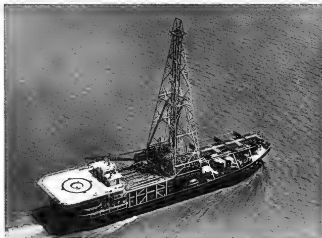
Cuss III—a floating drilling vessel. Courtesy Union Oil Co. of California.
