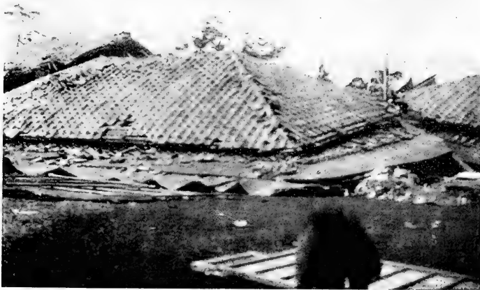
B. Collapsed houses in the villa of Prince Simadu, Kamakura.
