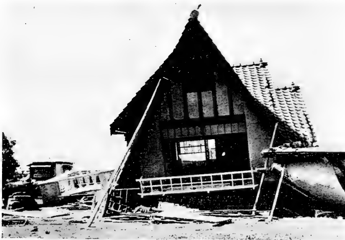
B. Collapse of a two-storied wooden house, Katase near Kamakura.
