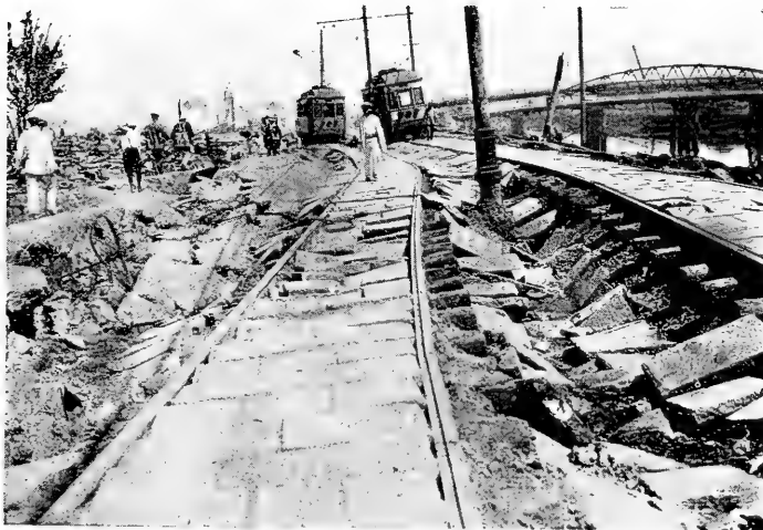
B. The central part of the City of Yokohama. Unequal settling down of the ground.
