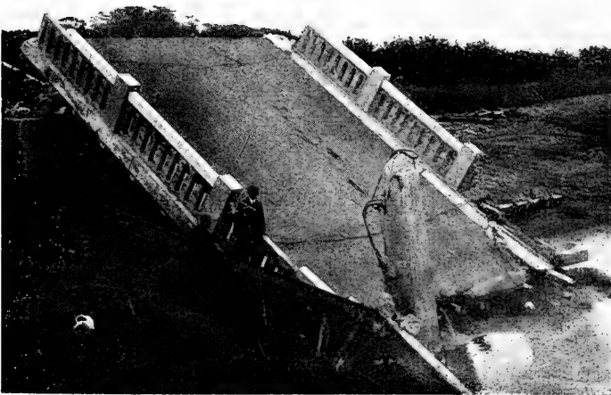
B. A part of Sakawa Bridge, Odawara. (Recently constructed; reinforced-concrete.)
