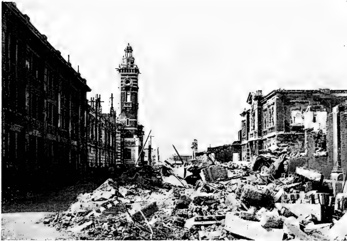
B. Hontyô street, near the port of Yokohama. Here the shock was next the severest in the city.
