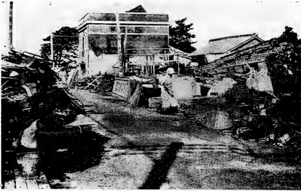
A. Ruins of the town of Hôdyô, Awa Province. A reinforced-concrete building in the back ground was intact.
