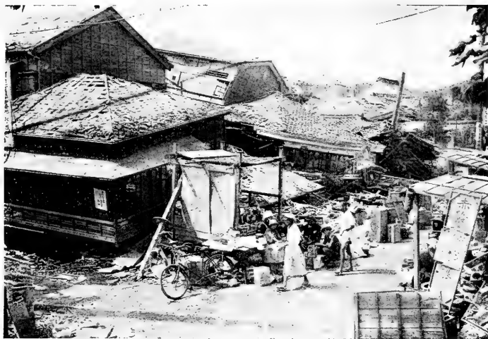
A. Collapsed wooden houses at Akasaka Mituke, Tokyo.
