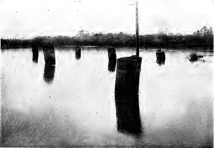
B. Roots of ancient bridge piers believed to have been buried for 700 years, but now exposed to the air. (Near Tirasaki.)
