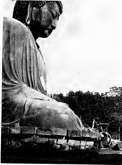
A. The bronze statue of Buddha, Kamakura. Displaced towards, and depressed in the right-hand side.
