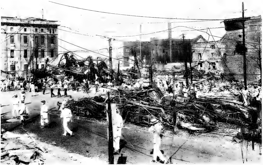
Fig. A. A scene in the business centre of Tokyo, after the shock and fire of the great earthquake of 1923: the skeleton of a burnt electric car in the centre. See p. 12.
