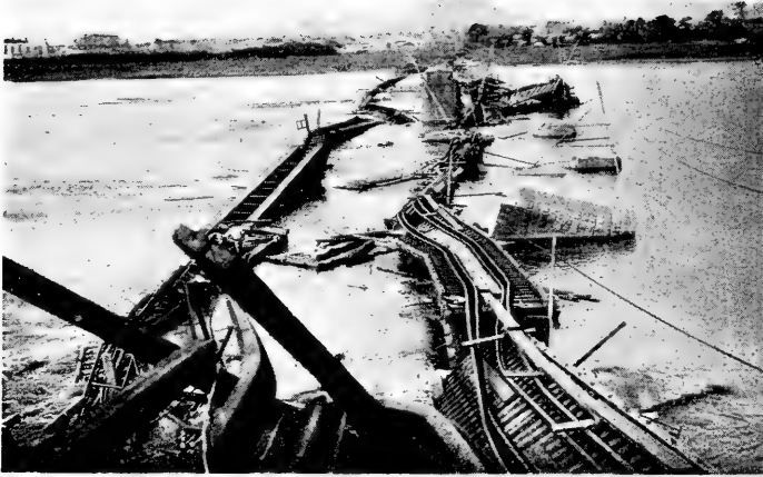
A. The complete destruction of the Banyúgawa railway bridge, near Hiratuka.
