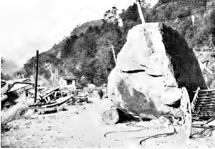
A. Damages in Yumoto, NE entrance of Hakone.
