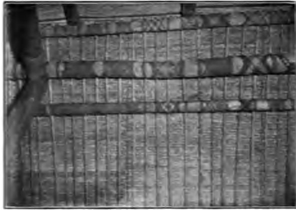
COCOA-NUT FIBER SENNIT WOUND AROUND THE ROOT-BEAMS OF A CHIEF'S HOUSE AT MBAU, FIJI.
