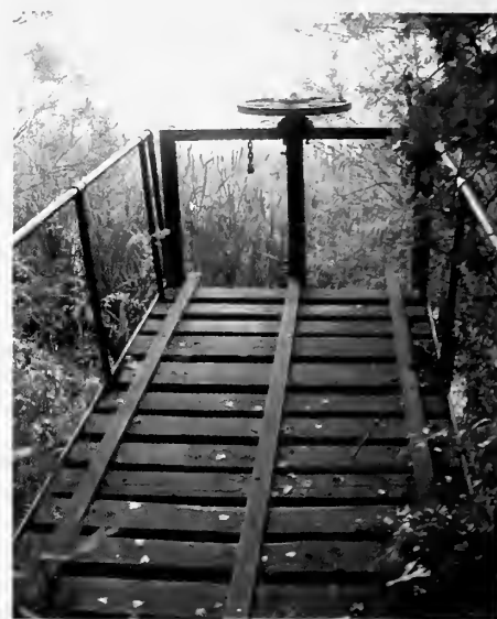
The sluice platform.
