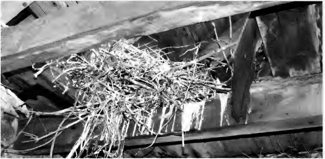
Plate 163. Common Raven nest in the roof of a ruined cottage, Sandwick, Orkney, May 2008 © C.J. Booth.
