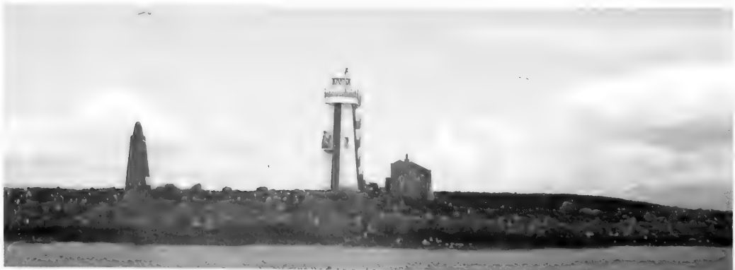
Plate 251. The old beacon lighthouse and warden's hut on Lady Isle are the only notable high points breaking an otherwise flat landscape suitable for breeding gulls, May 2012. © D. Grant
