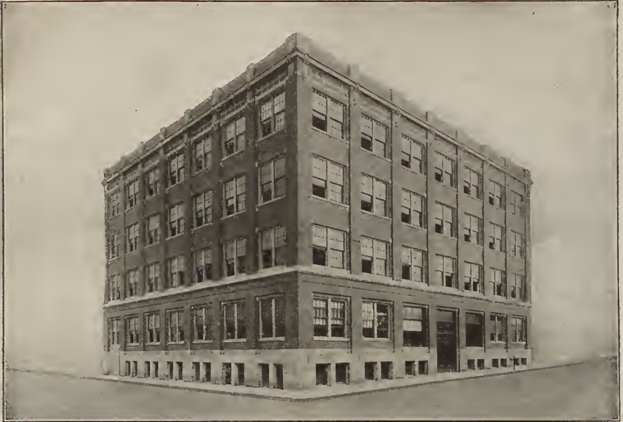
OUR NEW WINDSOR WAREHOUSE, ERECTED 1912
