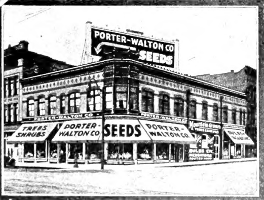
CITY STORE & OFFICES 42 WEST 1ST SOUTH
