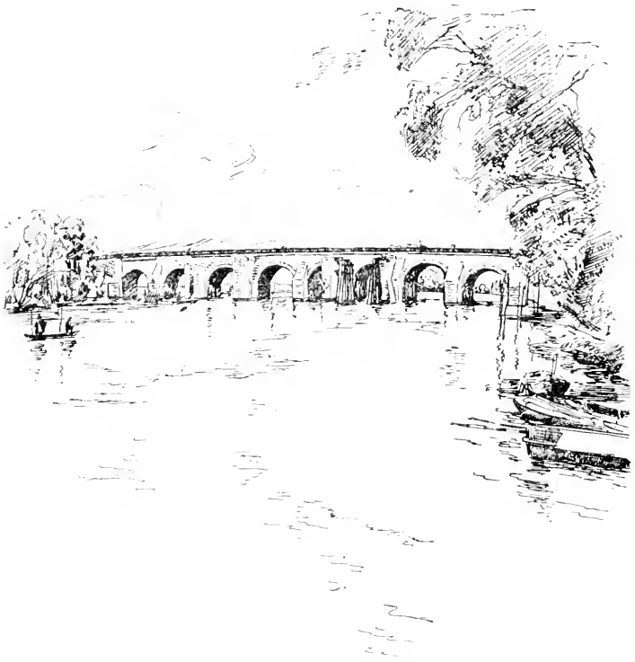
POISSY: THE BRIDGE.
