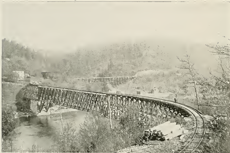
OLD B. & O. RAILROAD BRIDGE OVER THE CLARION RIVER
