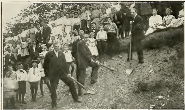
BREAKING GROUND FOR THE NEW DORMITORY.
